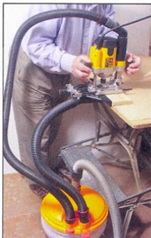
Using a router with two inlet hoses connected to the dust collector
